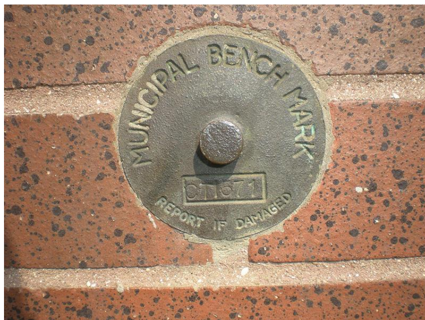
Fig. 4.5 City of Toronto benchmark disk in Canada.
